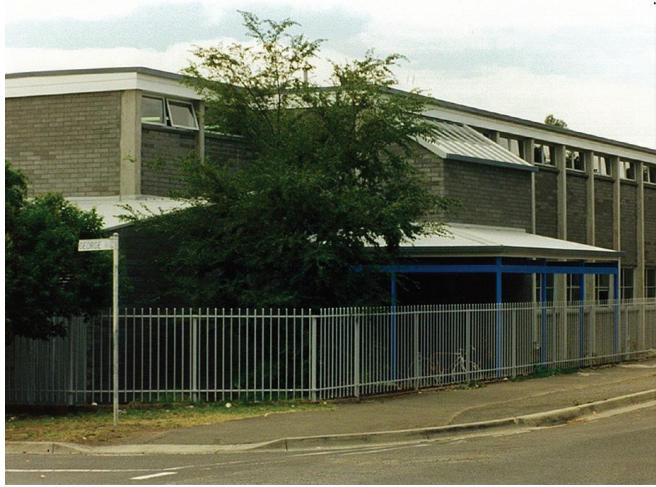
Maguire Wing Constructed
